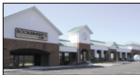
145. For Lease - Village Square in Christiansburg. 9,300 +/- SF retail/office space. New center, ready to build out for first tenants. Super location on Peppers Ferry Road across from New River Valley Mall. Don Moore or Roger Elkin 540.381.9000 540.982.0011
