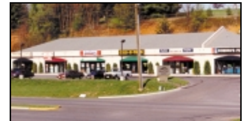
128. For Lease - 13,7000 SF of office/retail space on 1.22 acres with 890 SF currently available for lease. Located on Peters Creek Road. Chris Nelson 540.982.0011
