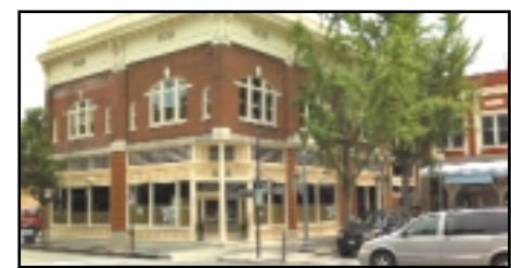
44. For Lease - 202 Market St. - Great professional office space located above 202 Market St. restaurant in the Historic Downtown Market area. Approximately 6000+ SF of space for single or multi-tenant use. Numerous offices already in place but could be redesigned. Brick outer walls with hardwood floors throughout. Lynn Hall 540.982.0011
