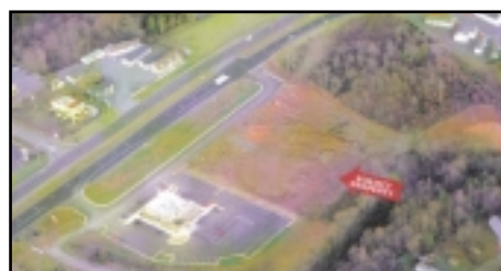
140. For Sale or Lease - US 460 East, Bedford County - 2 retail pad sites available between Applebee's and new Walgreens (site work in progress). Signalized intersection. Across from Wal-Mart Super Center. Ground lease, build to suit and land purchase available. High traffic count on major highway. Ideal for fast food restaurant, auto related store, C-store, or family-style restaurant. George Lupton 434.455.2306
