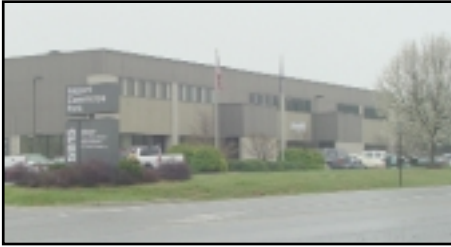
13. Roanoke, VA - Airport Commerce Center - Office/warehouse space for lease located near Roanoke airport. Ed Hall or Stuart Meredith 540.982.0011
