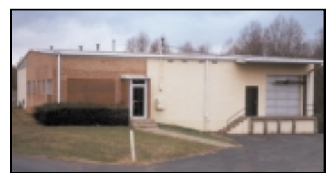
91. For Lease - 5,024 SF industrial building in excellent location. 1.66 acre sit allows for expansion. Paved parking area. Fully heated and cooled. +/- 1,000 SF office and the balance is shop space. $385,000. Chris Gentry 434.237.3384
