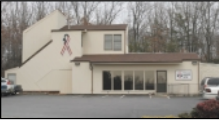
62. For Sale or Lease - 4,500 SF former medical office, Sheffield Drive across from K-mart. Zoning also allows retail use. Norman Moon or Chris Gentry 434.237.3384
