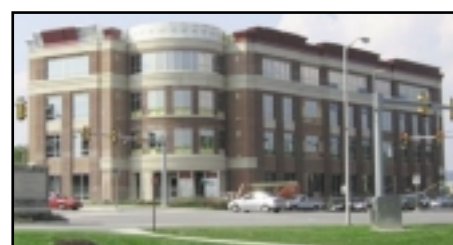
9. Blacksburg, VA - University Gateway Center - 80,000 SF office and retail building. Tommy Hendrix 540.982.0011
