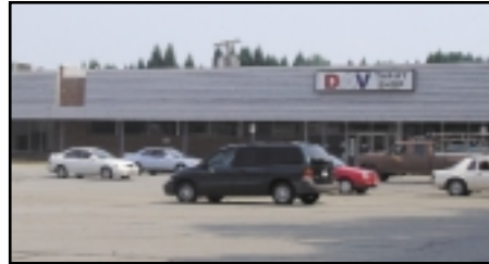
103. For Sale - Parkside Plaza Retail/Office building for sale in southeast Roanoke. 2,260 - 17,200 SF. Located on Route 24. Stuart Meredith or Ed Hall 540.982.0011
